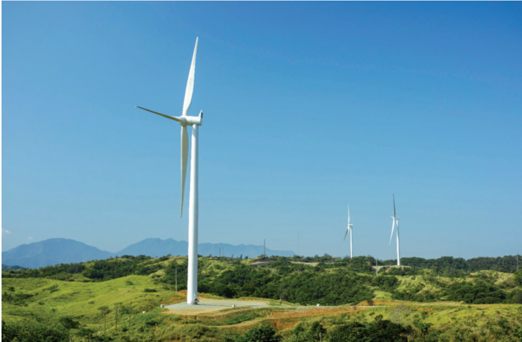
The 81 MW Caparispisan Wind Energy Facility. Photo courtesy of North Luzon Renewables/AC Energy
