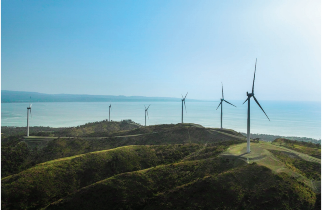
The 81 MW Caparispisan Wind Energy Facility, one of the renewable energy projects put up in 2014. Photo courtesy of North Luzon Renewables/AC Energy
